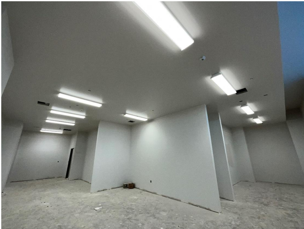
Locker Rooms Walls, Hard Ceilings & Light Fixtures Complete
