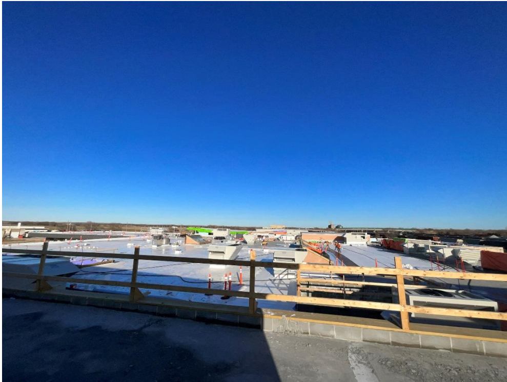
Light Weight Insulated Concrete Complete
