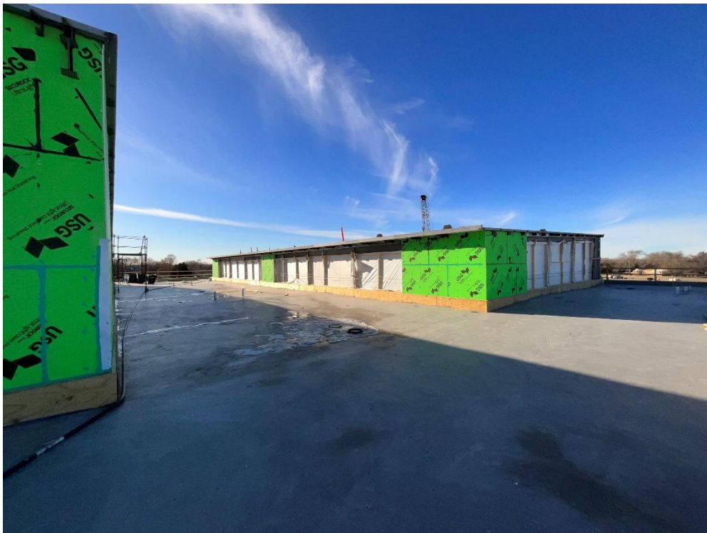
Light Weight Insulated Concrete Complete
